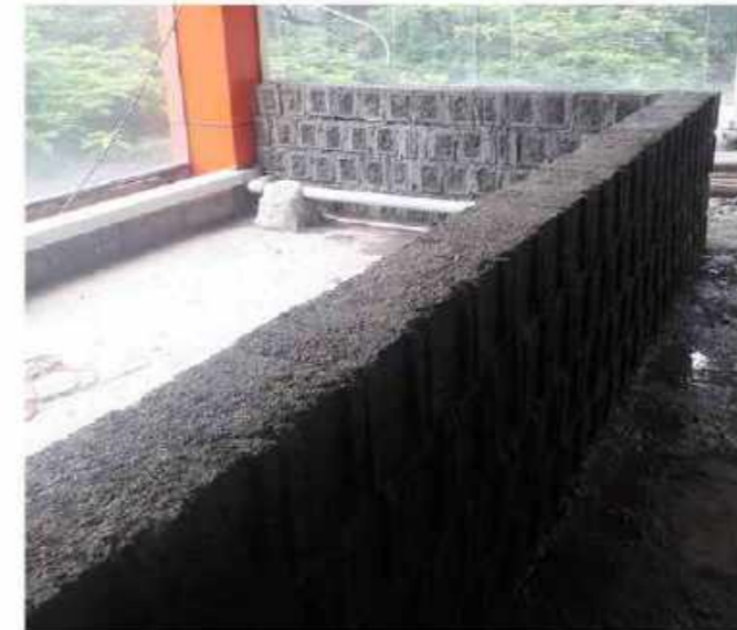
HOLLOW CONCRETE BLOCKS HAVE BEEN USED FOR THE BAR COUNTER TO GIVE IT A RUGGED LOOK
