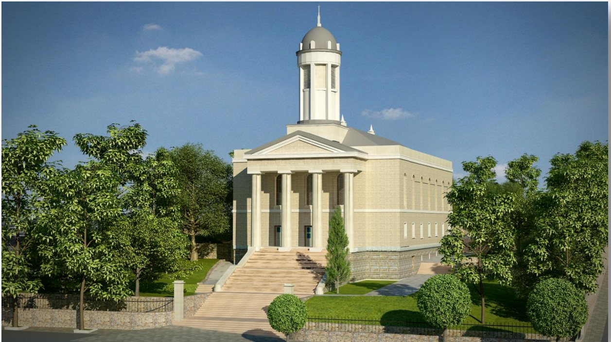
ST. George' s Church Renovation (U. S. A).
