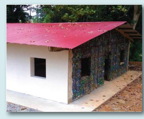
Discarded PET bottles can be used as bricks for construction of homes. In the island of Bocas del Toro in Panama, all the buildings are built using discarded plastic bottles.
