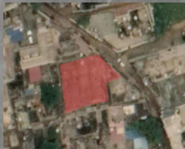
Site View @ Google Earth
