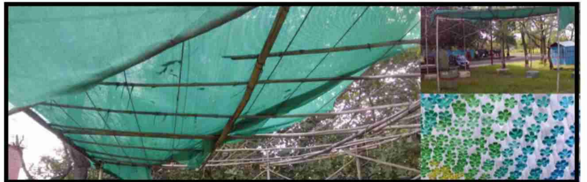
BAMBOO SHED, SIT OUT STRUCTURE BUILT FOR TECHNOSEARCH 2013
